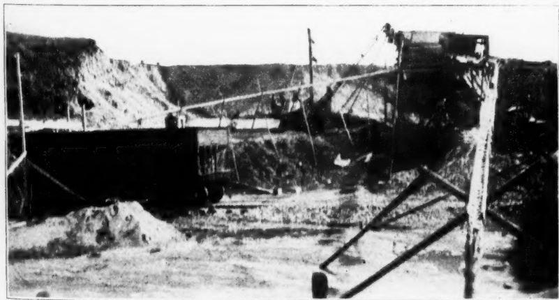
The Screening and Washing Plant.
